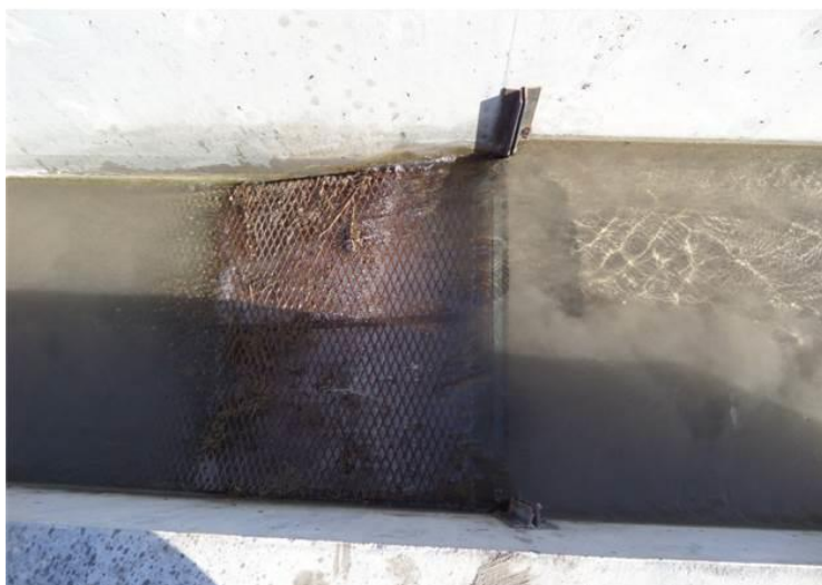
Figure 9. Fish barriers installed along restored stream channels in Rogers (upper) and Longstreet (middle) springs. Lower panel shows installation of removable plates and grate. Ash Meadows National Wildlife Refuge, NV.
